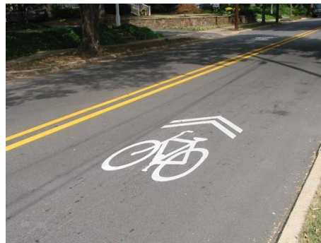
Figure 18: Shared Lane Marking in the center of a travel lane on Saint Mary's Street, Raleigh
